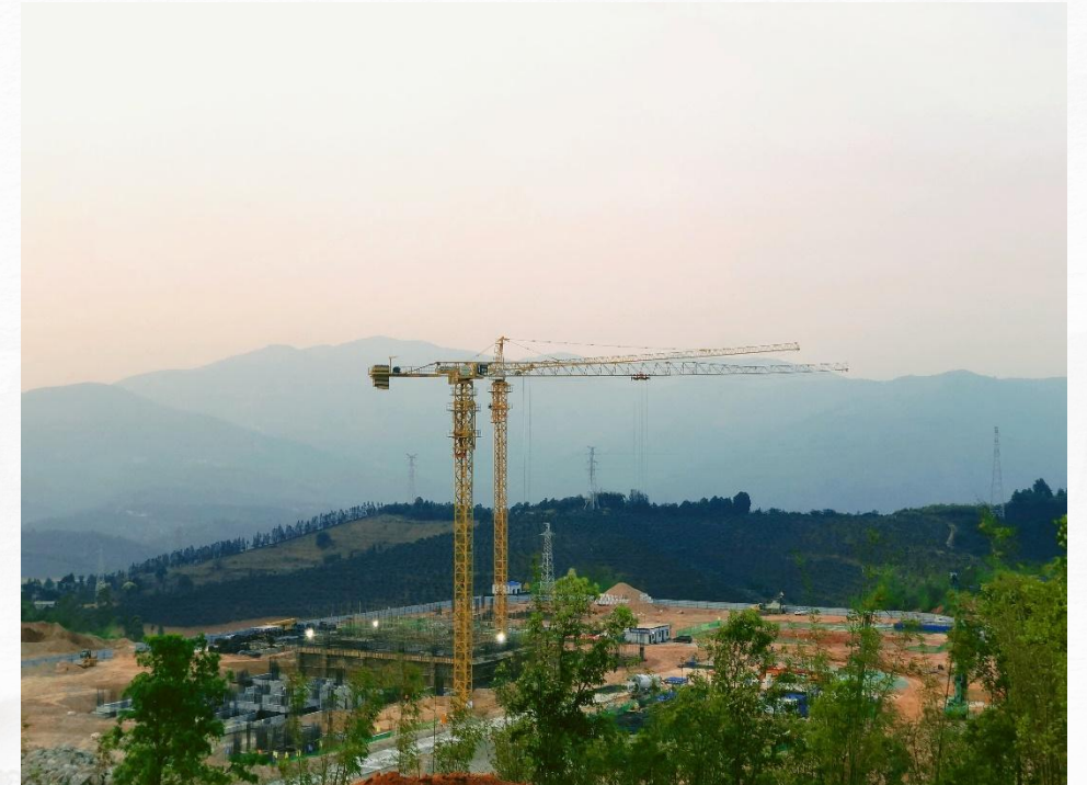
Jinghong Jiasheng WTE Facility
